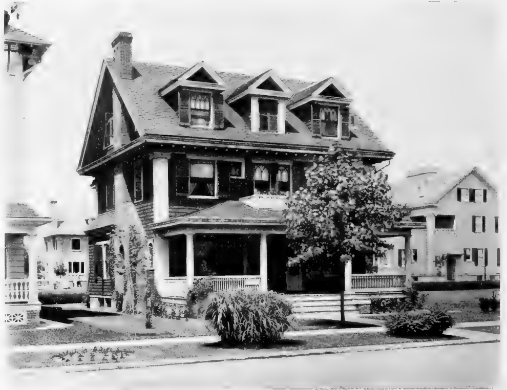
1—The House Built for Mr. Dean Alvord of Brooklyn, N. Y., can Stand Comparatively Alone, for it was Designed with That Intention
